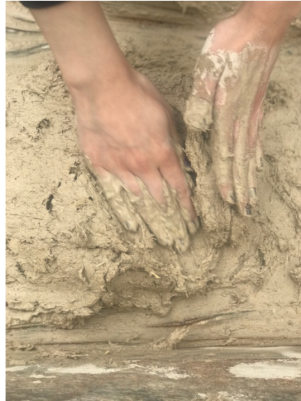
Fig. 35: Mixing earth materials
