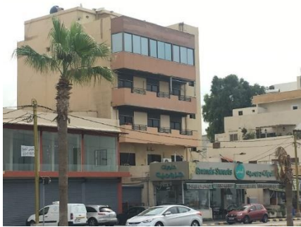
Figure 5.2.9. Balcony observed surrounded by 2 walls, Source: Author
