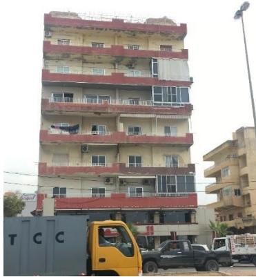
Figure 5.2.11. Balconies observed surrounded by 2 walls, Source: Author
