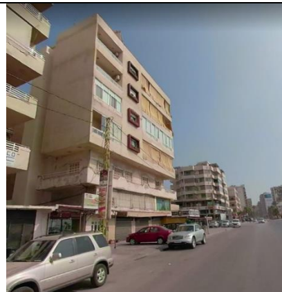
Figure 5.2.14. Balconies observed surrounded by 2 walls and 3 walls, Source: Author
