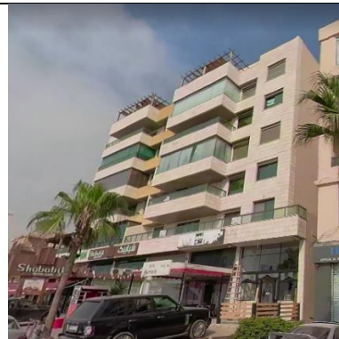
Figure 5.2.8. Balcony observed surrounded by 1 wall, Source: Author
