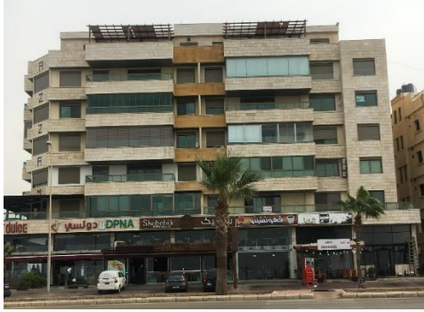
Figure 5.2.5. Balcony observed surrounded by 1 wall, Source: Author
