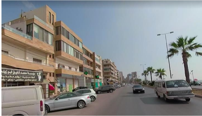
Figure 3.3.4. Glazed second and third floor in "Corniche El Baher" area. Source: Author
