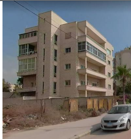
Figure 5.2.12. Balconies observed surrounded by 2 walls, Source: Author
