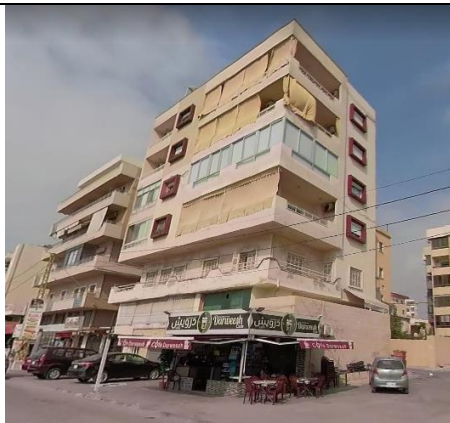
Figure 5.2.13. Balconies observed surrounded by 2 walls and 3 walls, Source: Author
