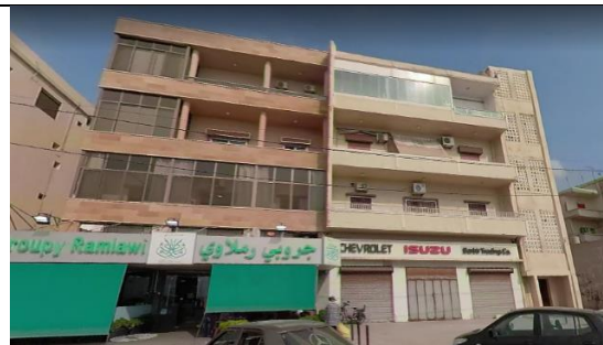
Figure 5.2.10. Balconies observed surrounded by 3 walls and 2 walls, Source: Author
