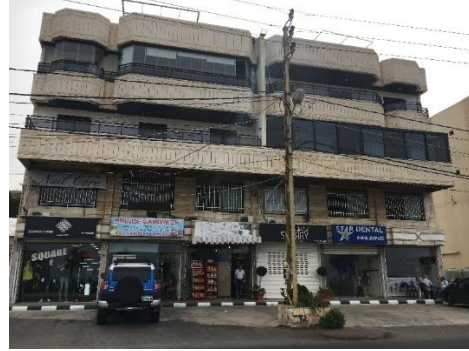
Figure 5.2.6. Balconies observed surrounded by 1 wall and 2 walls, Source: Author
