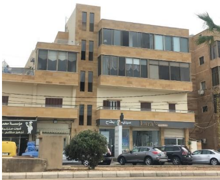
Figure 5.2.7. Balconies observed surrounded by 1 wall and 3 walls, Source: Author
