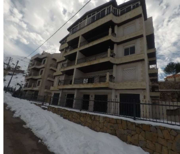
Figure 5.5 Picture showing building having the external envelope made of cavity wall with natural stone cladding. Taken on: January 28th 2020 . Source: Author
