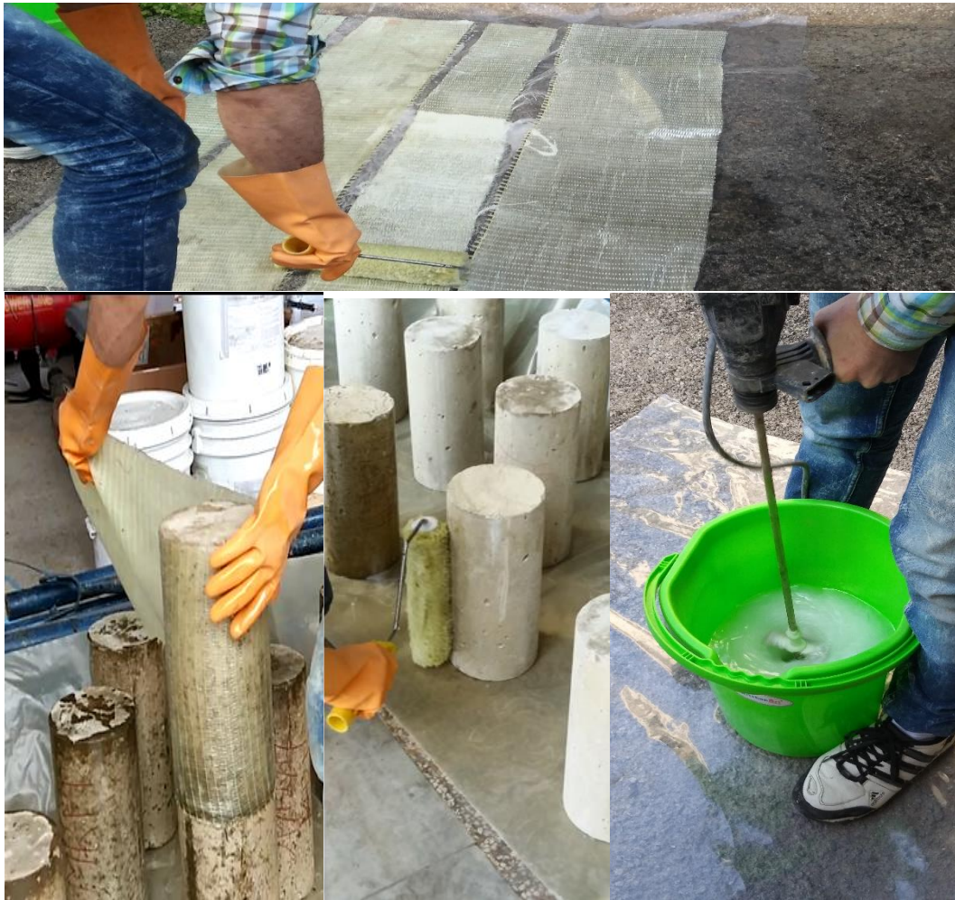
Figure III-3: Fiber reinforced polymer application technique
