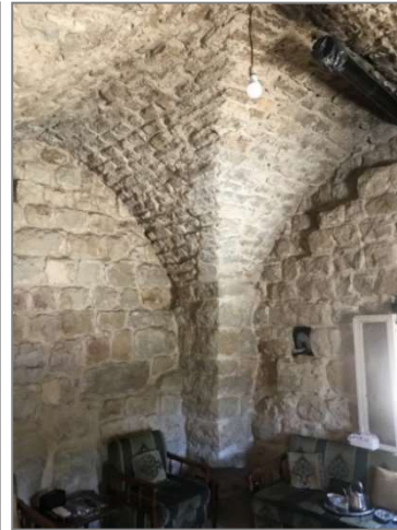
Figure 4.26 photo of the cross-vault structural base, Source: Author
