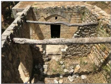
Figure 4.22 Photo for the post-lintel and barrel-vault roof, Source: Author
