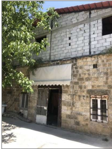
Figure 4.25 photo of the Liwan house with the additional construction added, Source: Author
