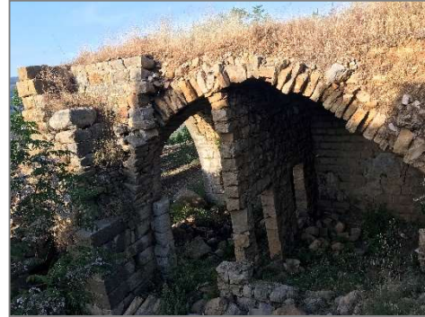
Figure 4.48 Photo of the existing Liwan house after destruction, Source: Author
