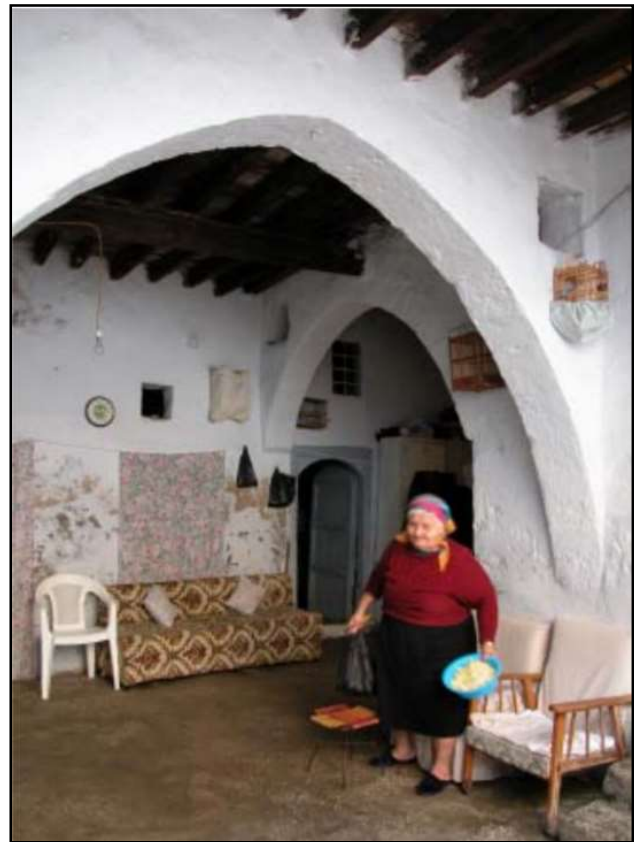
Figure 1.4 Liwan House in Tyr Having Inside and Outside Walls Rendered with Lime. Source: (Corpus and Euromed, 2003) Accessed 10-1-2021
