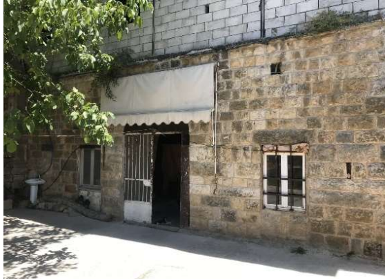
Figure 4.34 North-West Openings, Source: Author
