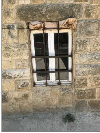
Figure 4.33 North-west openings that was a door and then transformed into windows, Source: Author
