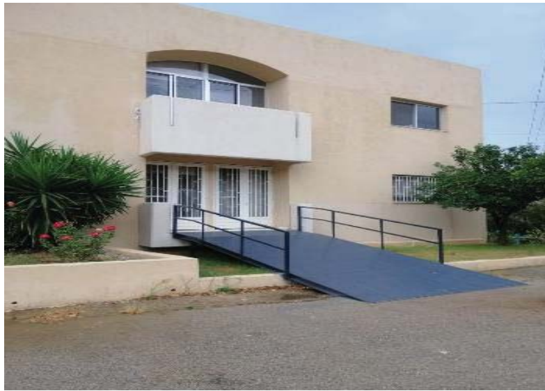
Figure 36: Building a ramp for the Covid-19 patients
