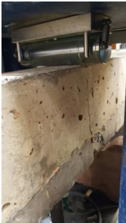
Figure 6. 3 - Spreader Beam for Loading
