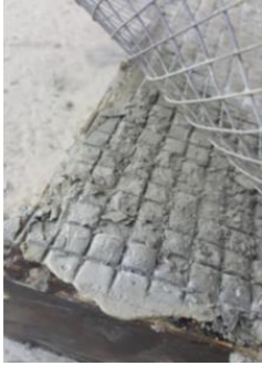
Figure 6. 11 - Steel mesh used to roughen the surface
