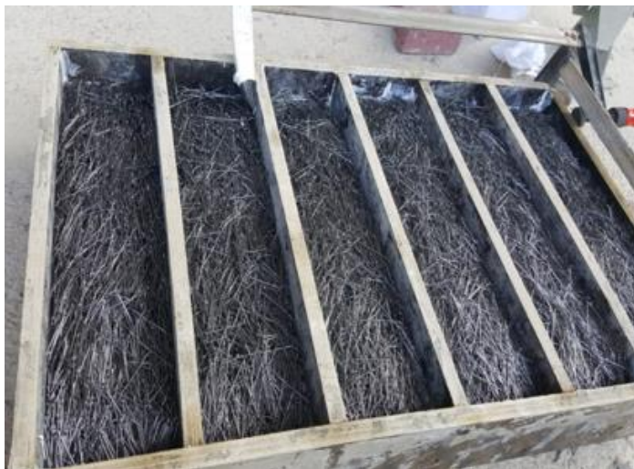
Figure 6. 21 - Elevated Formwork with SIFCON placed parallel
