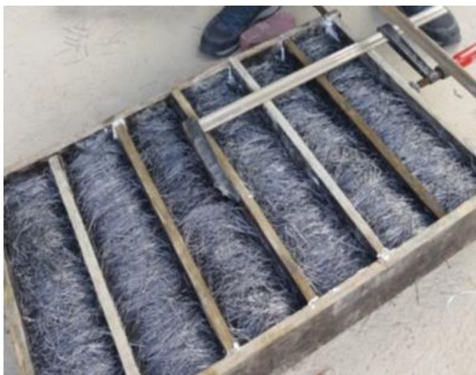
Figure 6. 22 - Elevated Formwork with SIFCON placed perpendicular
