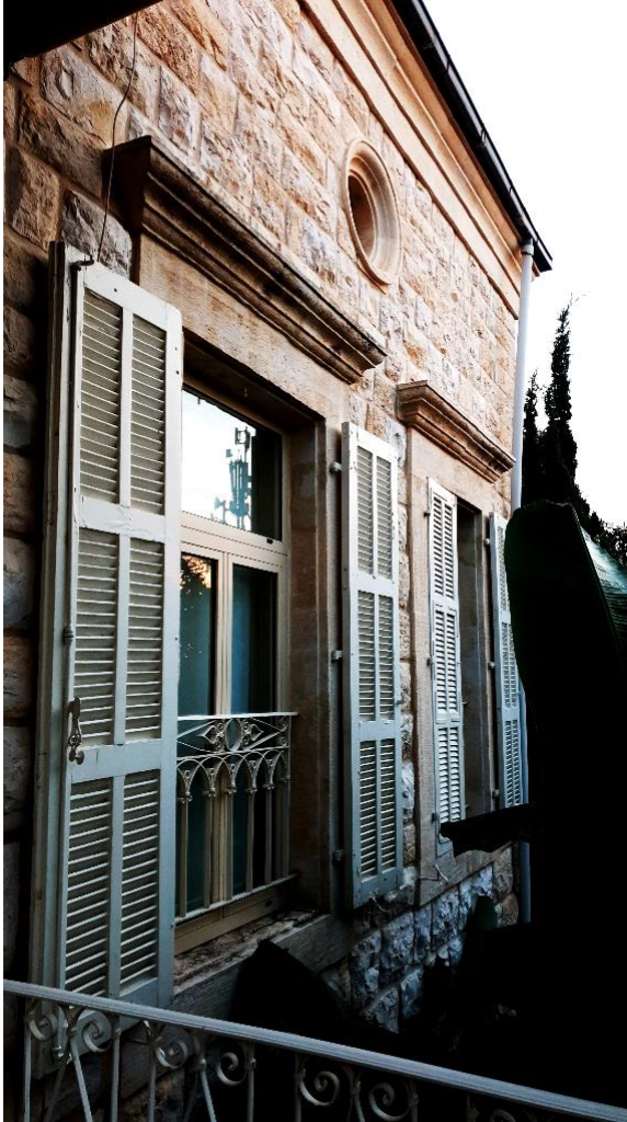
Figure 3.15: Windows and Small Opening, oculus of the North-West Elevation of the Old house- Ghazir.
